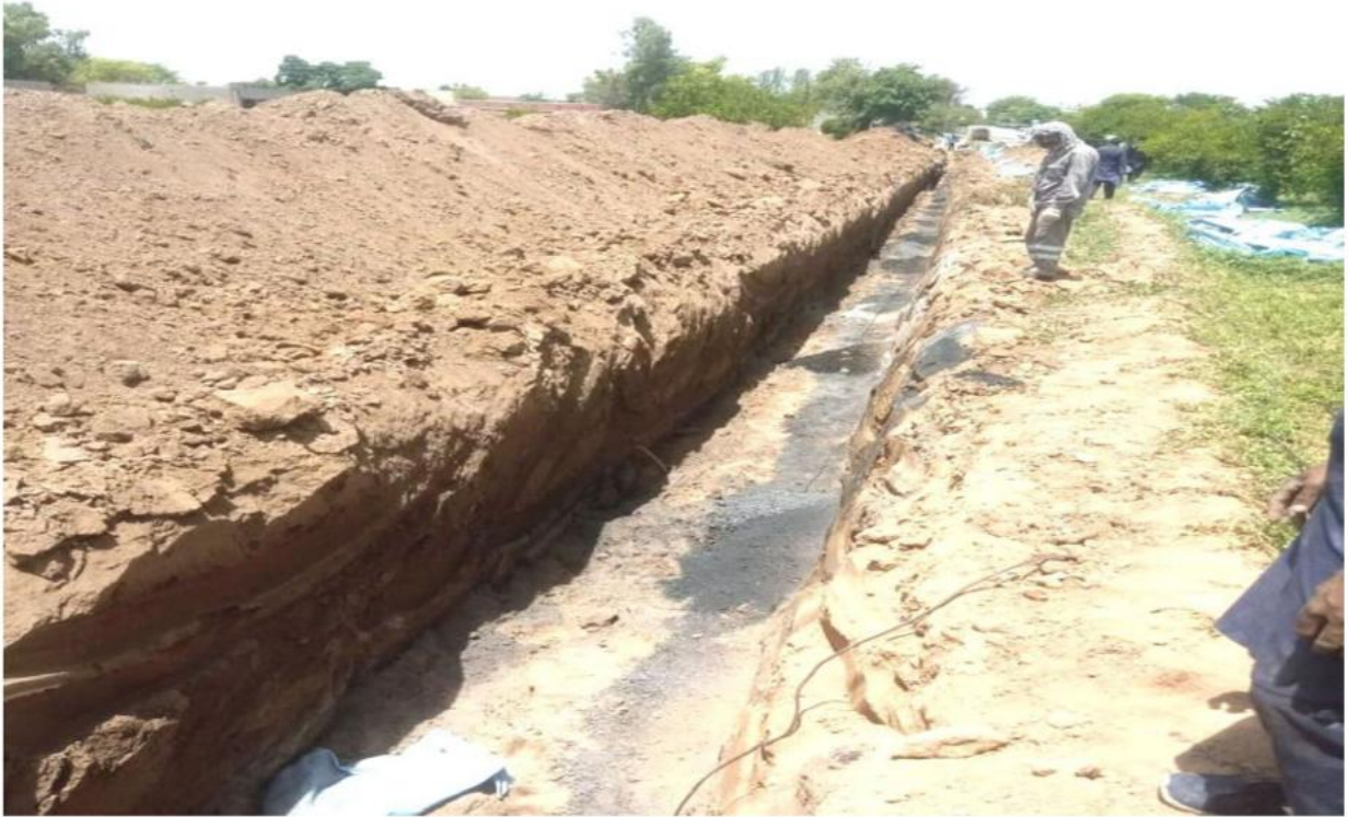
Figure 2.2: Laying of Horizontal Ground Bed
