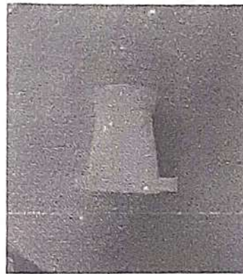
View-2 Where NRV is to be fixed
