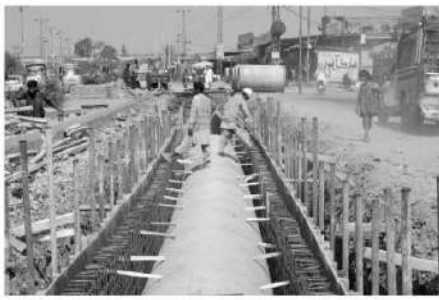
PESHAWAR: Workers install drainage pipes along Ring Road to improve the city's drainage system. —APP
